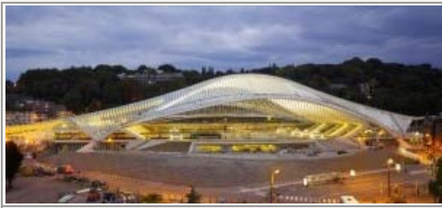
Liège-Guillemins TGV Railway Station
